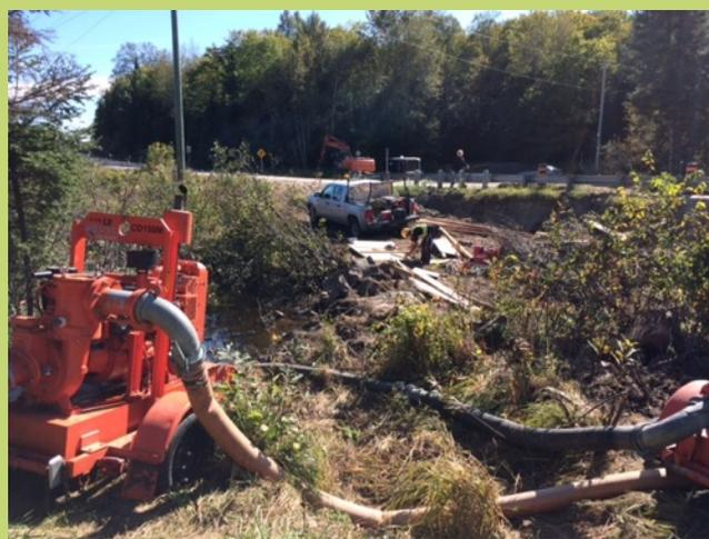
***As many of you may have noticed, there is major repair work going on along both sides of Highway 118 at Trapper's Trail, across from the mailboxes. Both ends of the culvert running under 118 are being re-built.***
